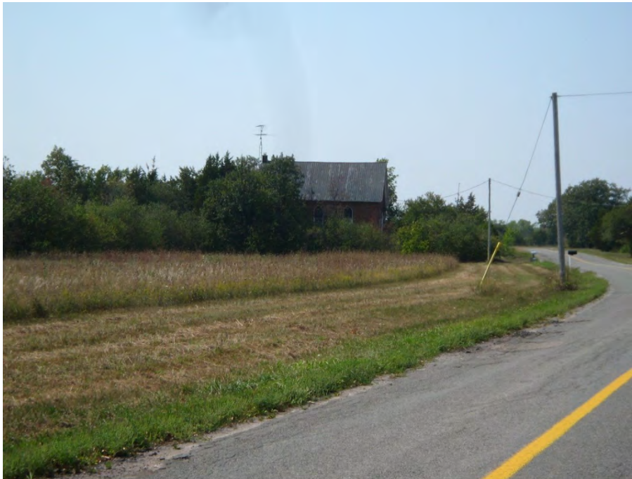
Plate 2: Bend in Long Point Road near Union G.M. Church
